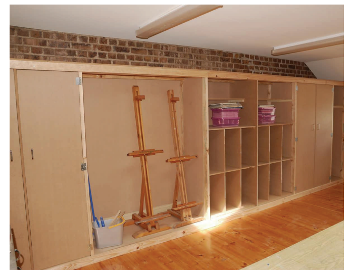
The cupboards are a new addition to the Mezzanine room at the Arts Company
